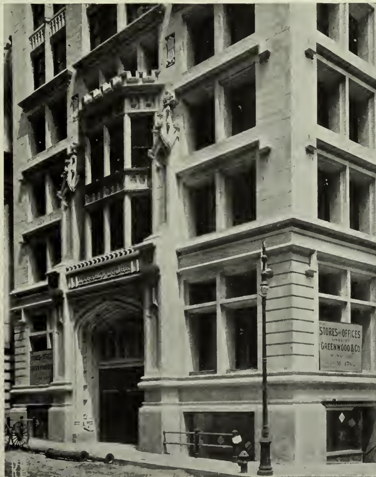
MAIN ENTRANCE TO LIBERTY TOWER BUILDING, NEW YORK CITY. Architectural Terra Cotta executed by Atlantic Terra Cotta Company. Henry Ives Cobb, Architect.
